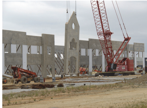
Construction of Shoppes at Meadow Creek
