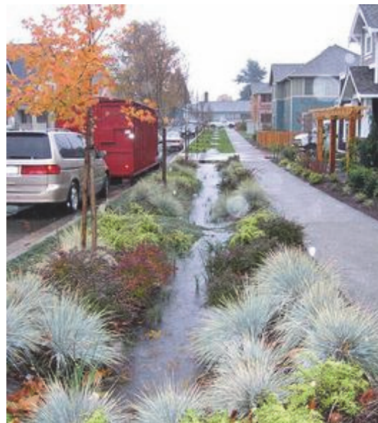
Example of a Bio-Swale
