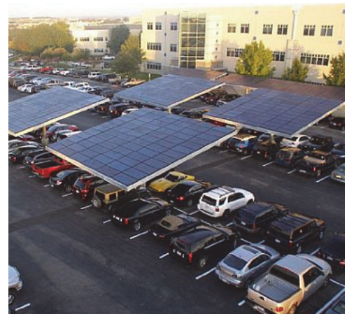
Solar Parking Lot
