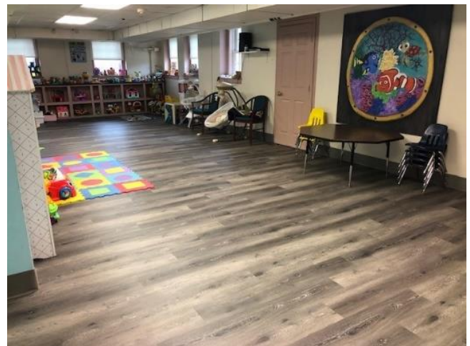
New flooring installed at the Family Center
